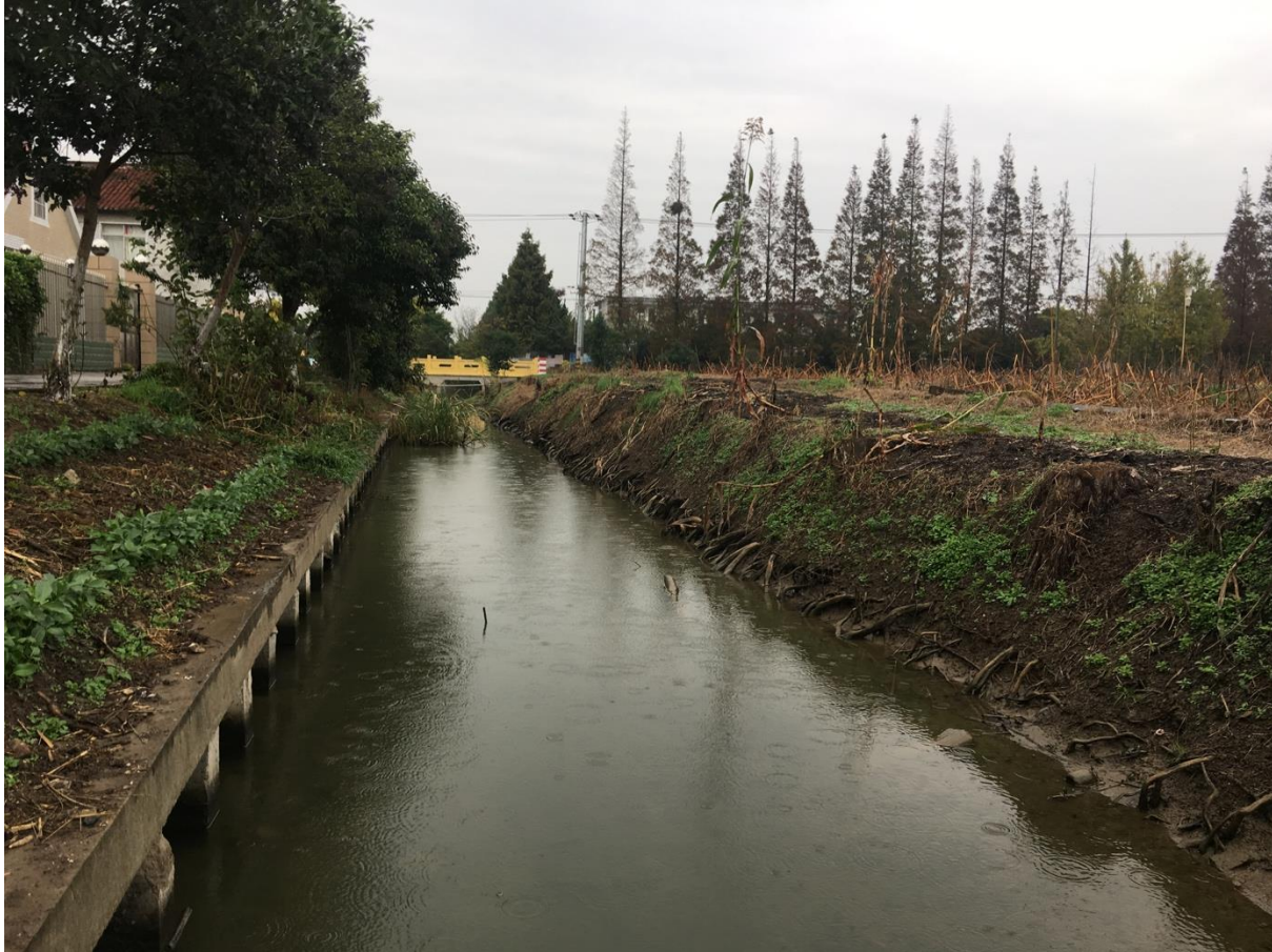
Figure 4: Trees were cut down and their roots remain by the riverbank
