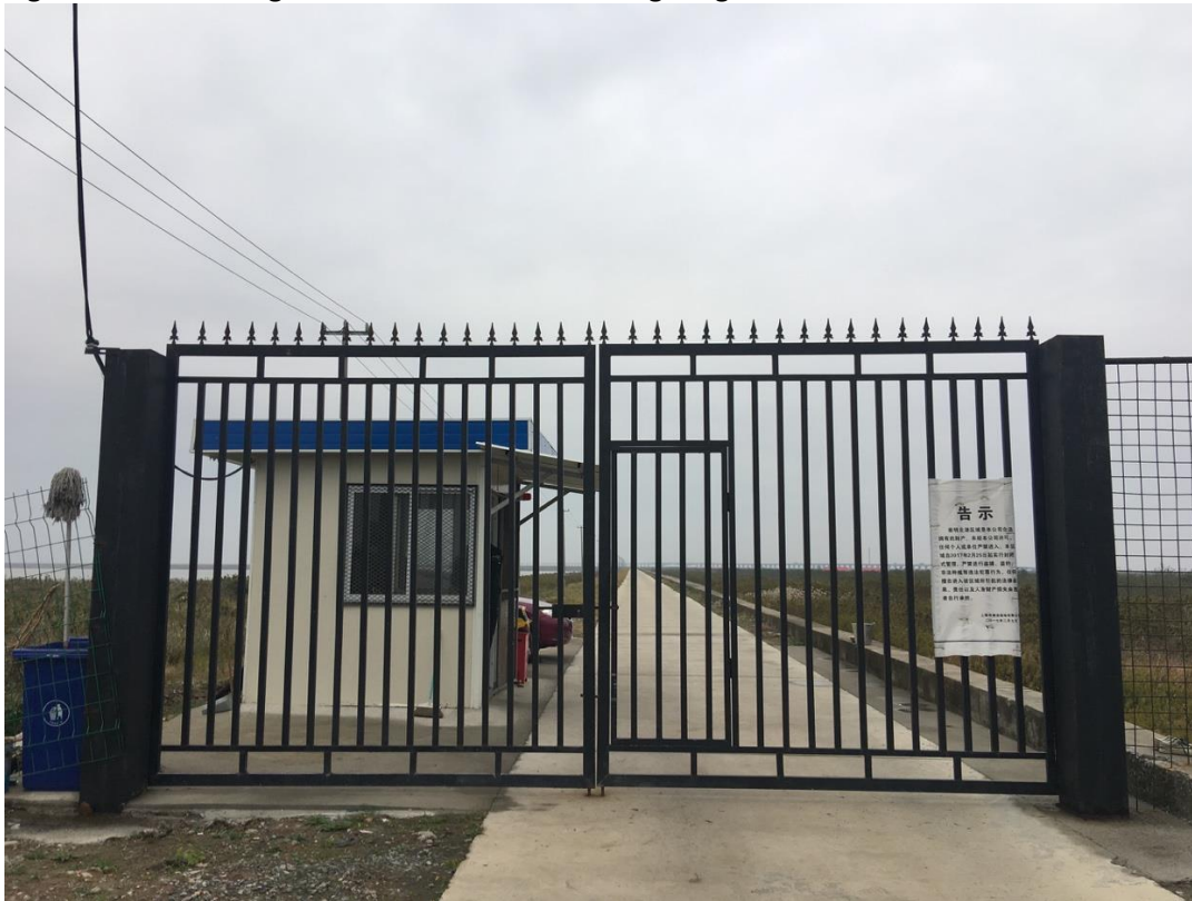
Figure 8: The metal gate at the entrance of Chongming North Lake
