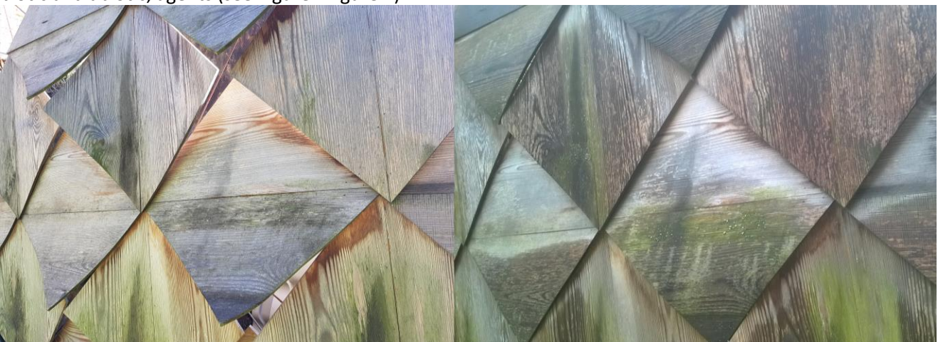
Figure 2: Responsive solid wood screen Ray 2 co-performing with relative humidity, algae moisture sorption and temperature. The responsive wood panelling is moderating micro-climate: either producing humid air flow through its warping and moisture evaporation in hot and dry weather or sorping and enclosing it in humid and cold situation. This is moderated by algae moisture sorption: larger warping when dry and hot, prevention of warping in opposite direction when it rains. (photos: Davidová 2018 and 2017)
