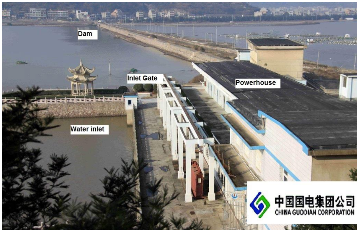
Figure 2-22 The powerhouse and the dam at Jiangxia Tidal Power Station (Image source: Chain Guodian Corporation)
