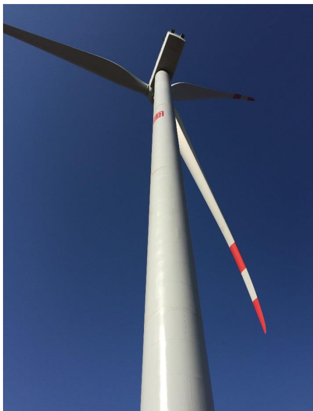
Figure 2-25 3,000 kW wind turbine
