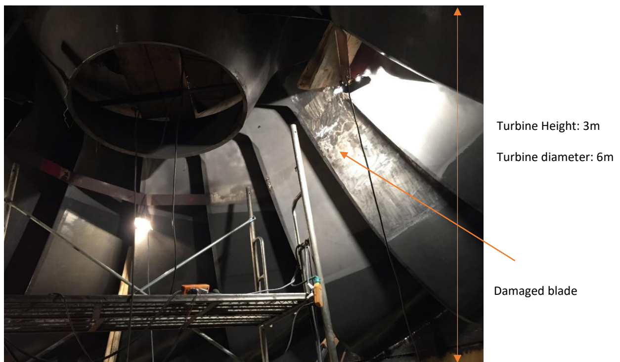
Figure 2-19 Repair of the damaged blades of the No.4 Francis Turbine
