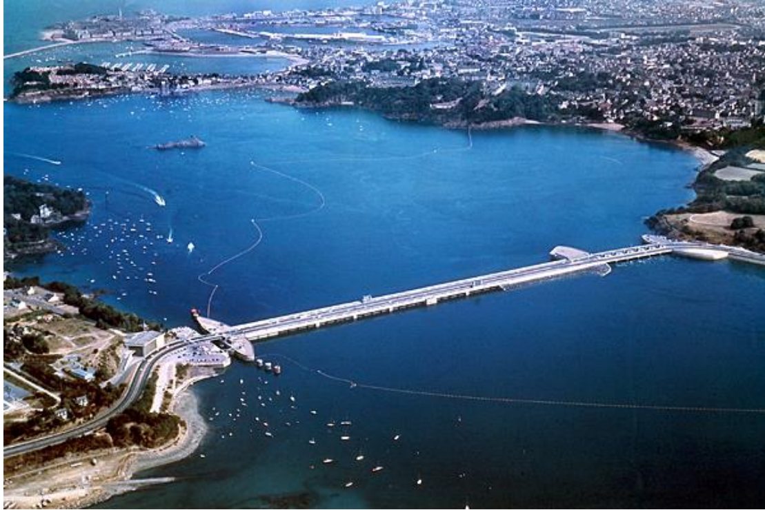
Figure 2-13 La Rance Tidal Power Station, France (Image Source: tethys.pnnl.gov. 2009)
