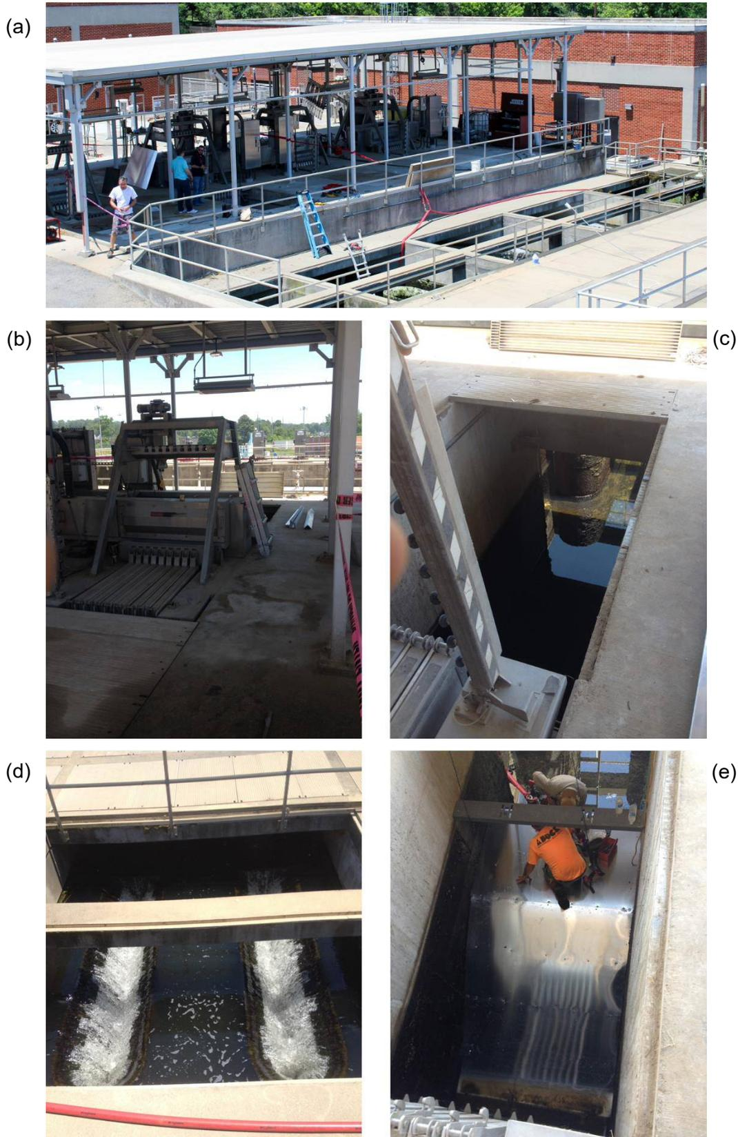
Figure 92. a) UV disinfection channels at RM Clayton. There are five UV canals in total of which three are in operation. Channel two is allocated for the turbine; b) non-immersed UV lamp housing of channel two (~2m above water level); c) downstream of UV lamp housing in channel two where the turbine is installed; d) UV channel effluent weir; e) installation of constriction
