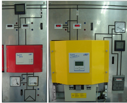
Fig. 6.3 NTUA equipment: PV inverter (left) and battery inverter (right)
