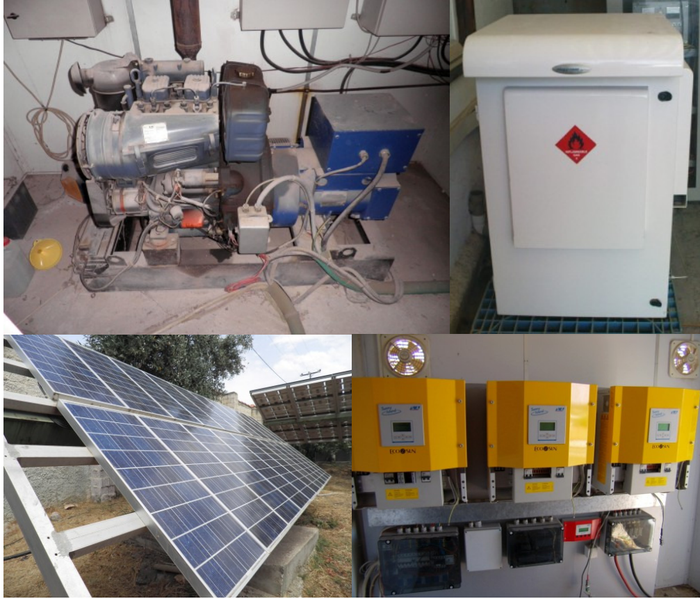
Fig. 6.5 CRES Diesel genset (upper left), fuel cell (upper right), photovoltaic (lower left) and battery inverters (lower right)
