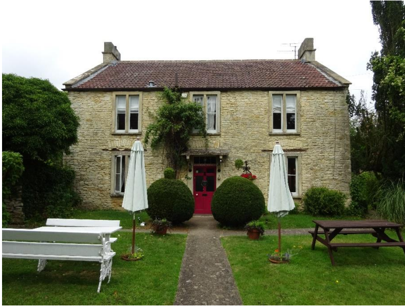
Fig. 15. Fosse Farmhouse (photograph by the author).
