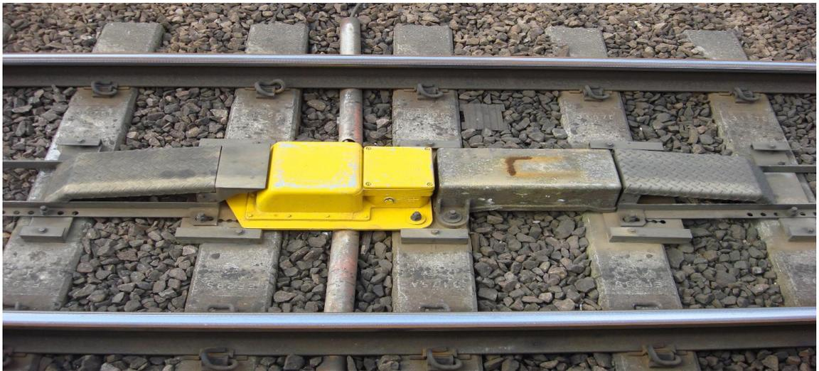
Figure 9: Automatic Warning System (AWS) track equipment (permanent magnet and electromagnet)
