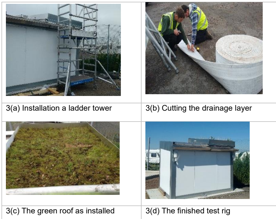
Figure 3. Green Roof Installation
