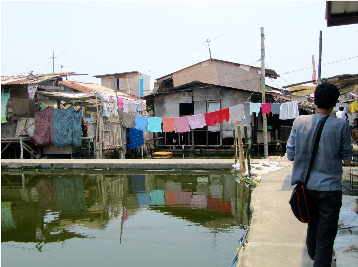
4. Del Rosario settlement, Valenzuela City, Metro Manila, yearly undergoing severe floods: the community is currently seeking to upgrade its settlement through reblocking (Photo: Giorgio Talocci).
