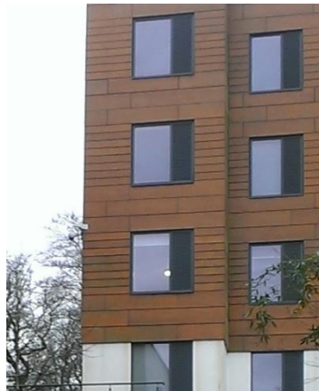
Figure 72. Facade with fixed louvers. MH.
