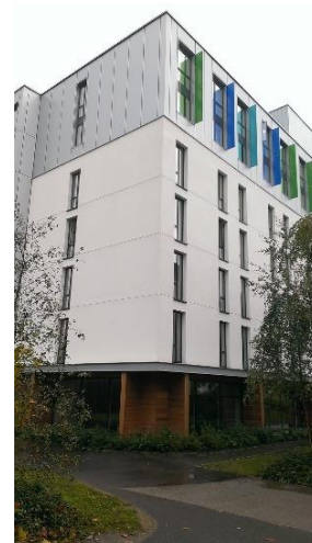
Figure 70. Full-height windows with shading panels. CC.
