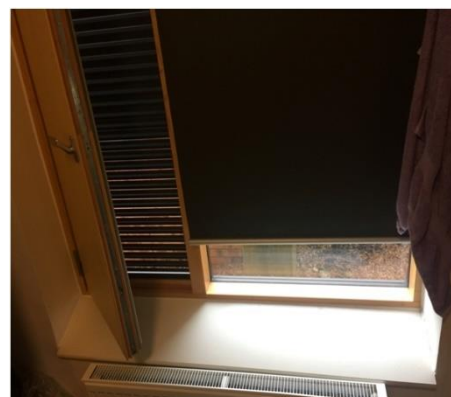
Figure 68. Compromise to reduce littering. MH.
