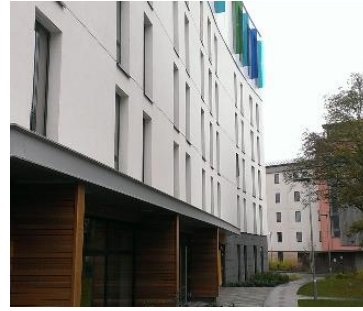
Figure 56. Recessed windows. CC.
