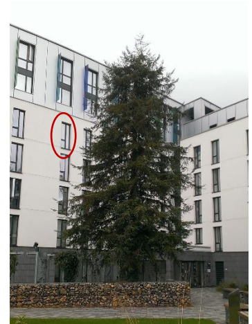
Figure 85. Narrow, full-height CC windows
