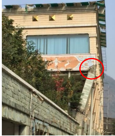
Figure 5.11: Detail of the column analysed as a singularity element given its location in the junction between the building blocks presenting different elevations.
