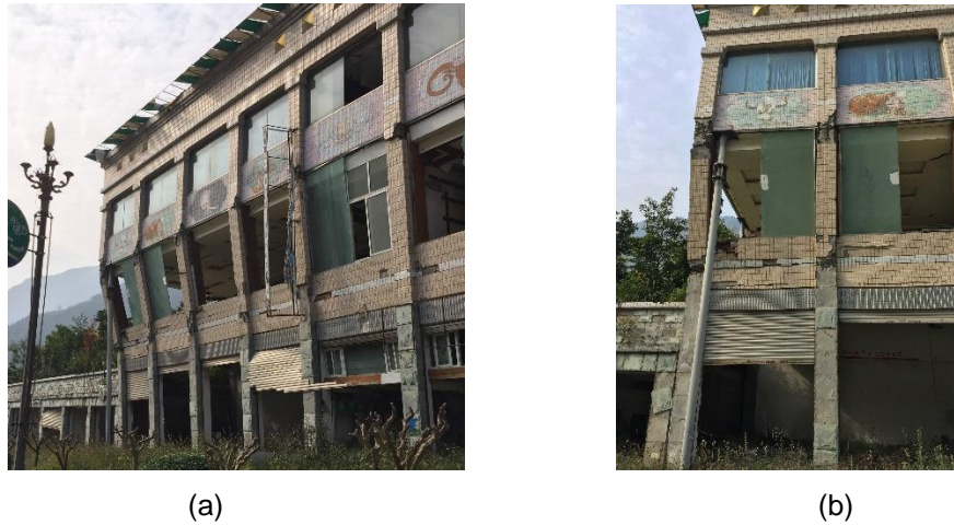
Figure 5.5: Photographic material regarding Beichuan Hotel, as-built configuration as to December 2016 field trip with detail of façade (a) and masonry infills (b).
