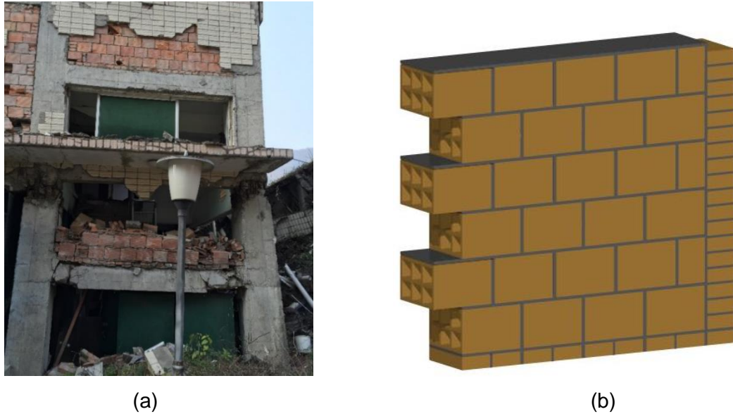
Figure 5.9: Masonry infill details for police station building in Old Beichuan (a) and virtual representation (b).
