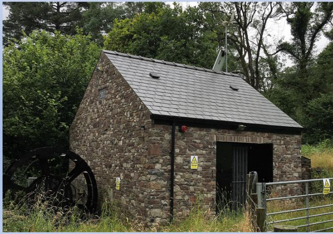
Image: Micro-hydro turbine 'house' with micro-wind turbine and waterwheel
