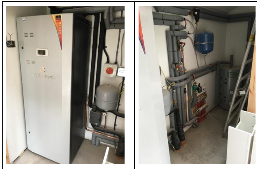
Figure 7.16. Domestic Ground Source Heat Pump (GSHP) Condenser (left) and necessary plumbing (right) Source: Author
