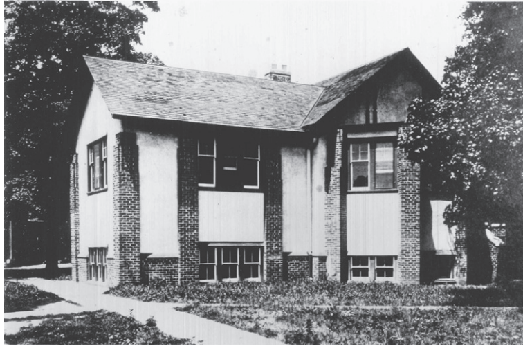
Figure 3. Park Ridge Public Library, in an Arts and Crafts idiom (opened 1913). Source: Courtesy of Park Ridge Public Library.
