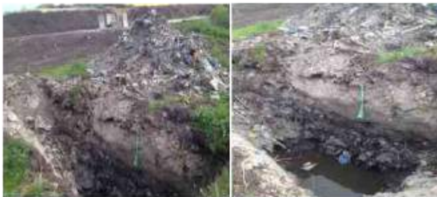
Figure 13. Test excavation (photo May 2016) on top of Stage 1 Skårup Landfill
