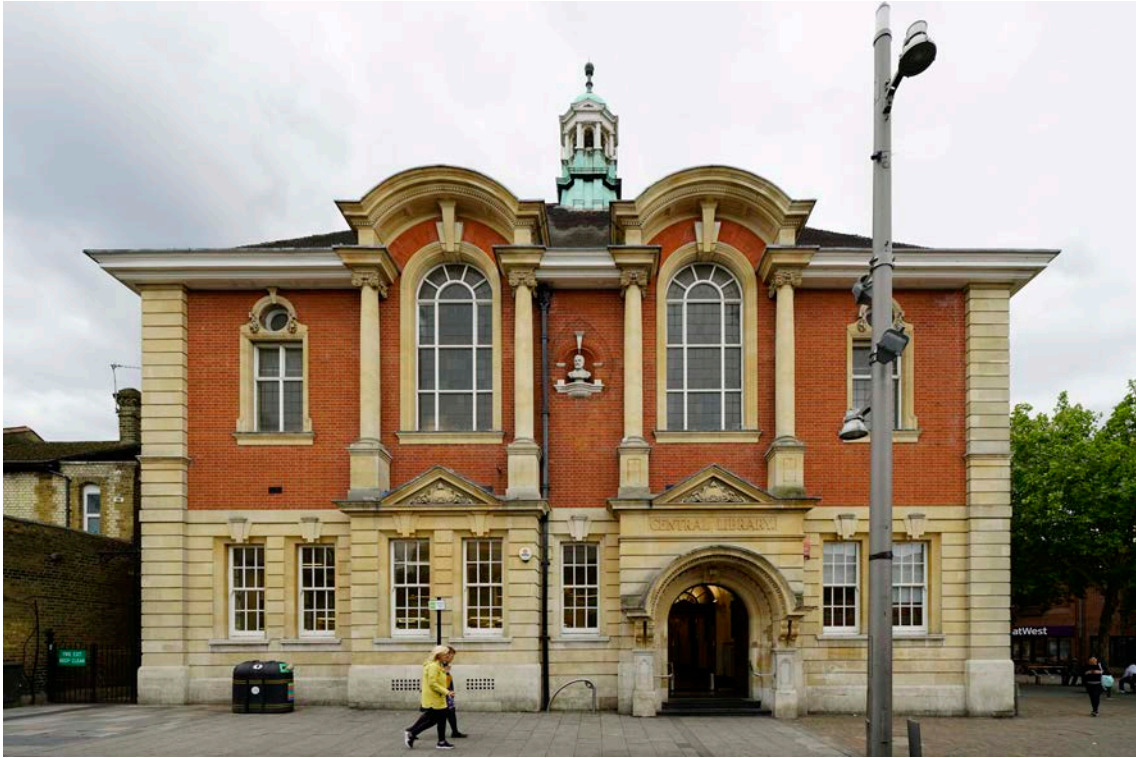
Figure 2. Walthamstow Central library Exterior (OP)
