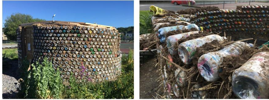
Fig. 11 Ecobricks used in a community garden project - Bwyd Bendigedig Port / Incredible Edible Porthmadog, UK ©Lizzie Wynn, 2020
