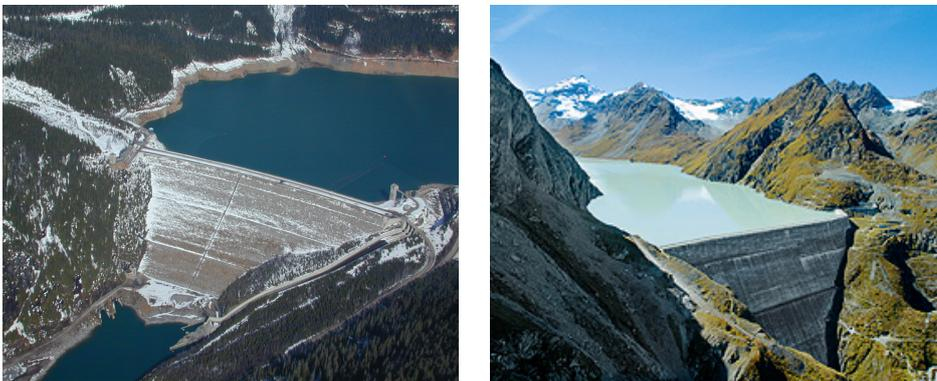
FIGURE 2.2: Embankment dam; Mica Dam, Canada (Christensen, 2019) on the left and Gravity dam; Grande Dixence, Switzerland (Grande-dixence, 2019) on the right.
