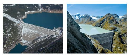
FIGURE 2.2: Embankment dam; Mica Dam, Canada (Christensen, 2019) on the left and Gravity dam; Grande Dixence, Switzerland (Grande-dixence, 2019) on the right.
