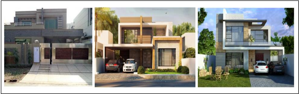
Figure 2.42 Glimpse of Pacca (brick-concrete) houses of Punjab, Source: Author
