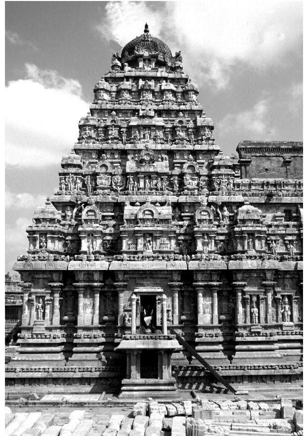
12. Airāvateśvara temple, Darasuram (Tamil Nadu), mid-twelfth century, a five-storey ( pañcatala ) vimāna . Unlike the equivalent temple in the Samarāṅgaṇa, here the kūṭa , pañjara , and śālā pavilions crowning the first and second tiers are two-storey ones ( ṣaḍvarga , ‘of six divisions’), i.e. equivalent to the entire śālā aedicule of Figure 6 (photo by Gerard Foekema).
