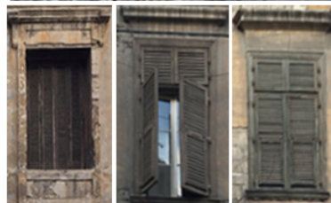
openings frame are made of wood with external wooden light shutter
