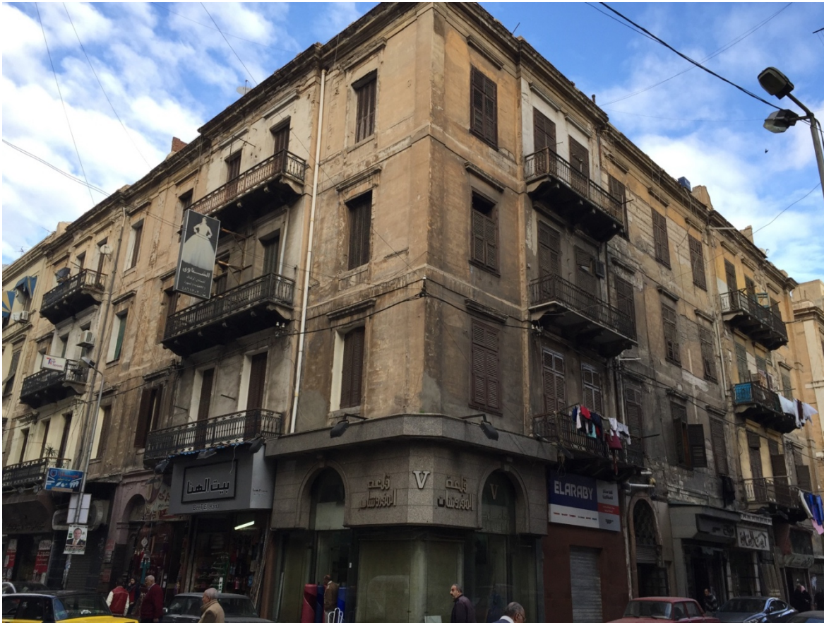
Figure 5-1 case study building, source: the researcher
