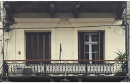
The handrail is made of steel work with a wooden parapet
