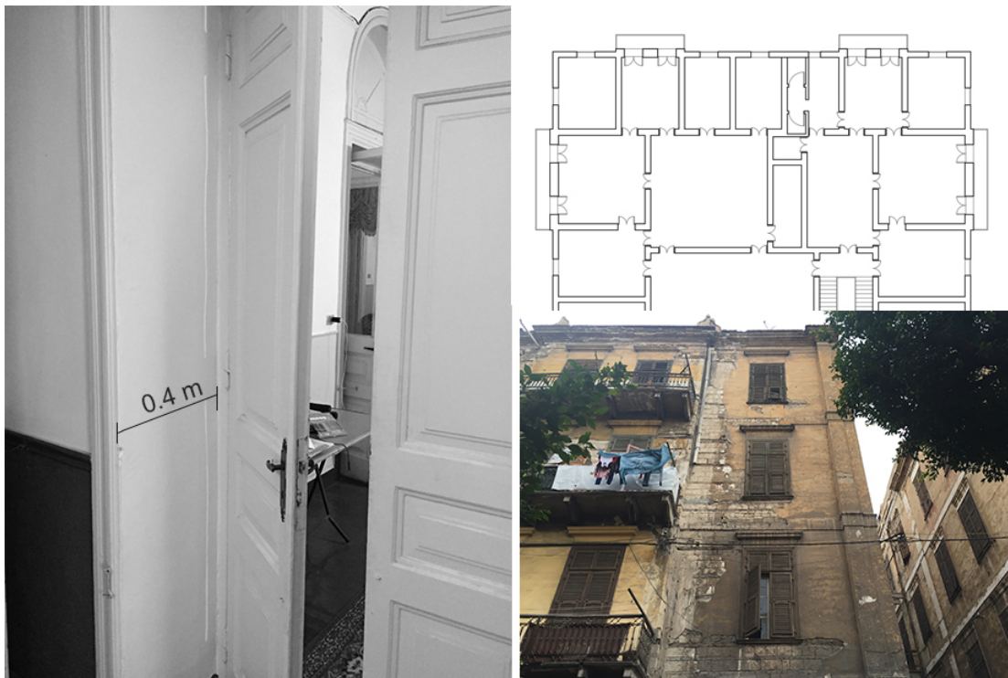
Figure 5-16 the thick walls of the building, source: the researcher
