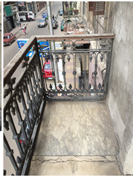
The handrail is made of steel work with a wooden parapet
