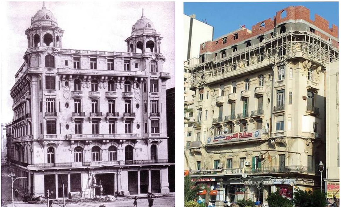
Figure 2-54 new addition to Majestic hotel (Forster, 2014)
