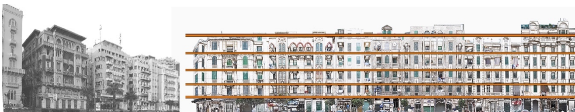
Figure 2-49 The stories heights form a datum within the heritage context
