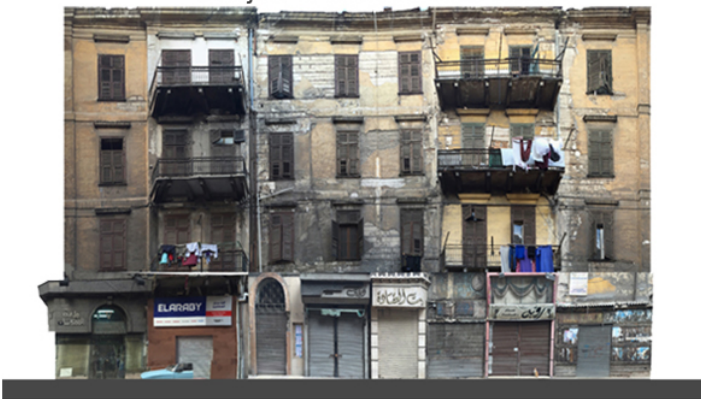
Sizostreis street Facade
