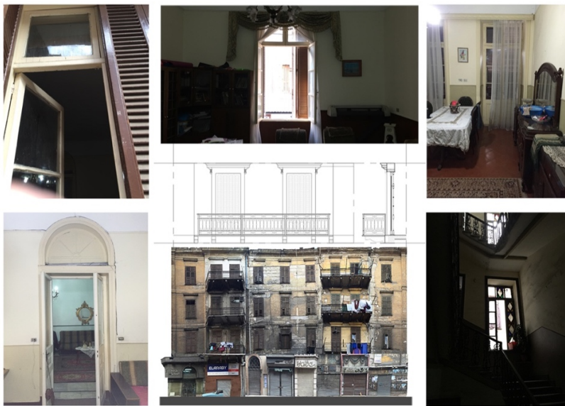
Figure 5-29 external and internal opening types
