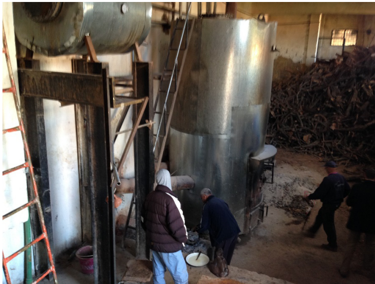
Figure 4 The improved furnace at hammam al Karam, Marrakech (Photo taken in January 2015 by Dr Magda Sibley)
