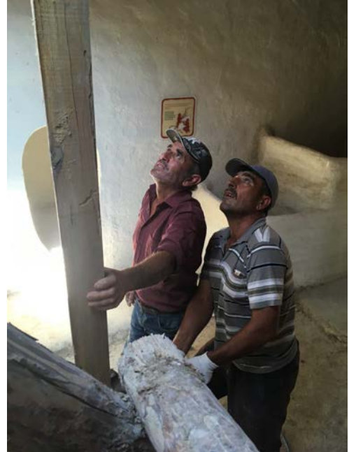
Figure 4: Ahmet Bülüç and Zekeriya Sivaz fixing roof of a model house (Photo by Berkay Dinçer).
