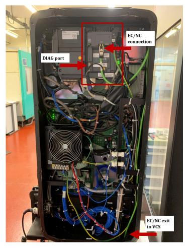
Figure 3.3. FCU7 installation and Ethernet cable routing
