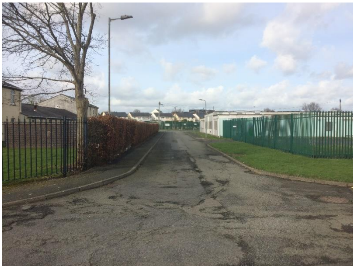
Figure 3.3d: entrance to the site
