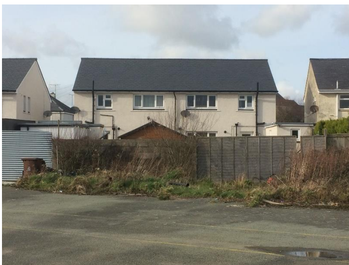
Figure 3.3e: adjacent properties backing onto the site
