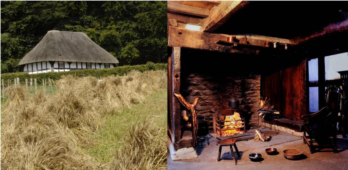
**Figure 3: Aberndowydd Farmhouse, a timber-framed thatched farmhouse built c.1678. Originally an open hall design with central fire open to the roof, the stone-backed fireplace and timber-framed chimney later additions c.1708 (National Museum Wales).**
