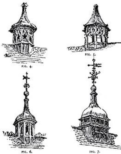
**Figure 15: Various smoke louvres on Medieval Halls, showing the similarity in the design for the smoke apertures of chimneyless buildings (Shuffrey 1912, 7).**
