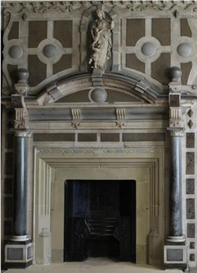
**Figure 21: Tudor fireplace in the Renaissance style, reduced and a 19th C cast iron grate inserted for burning coal, at New Hardwick Hall.**
