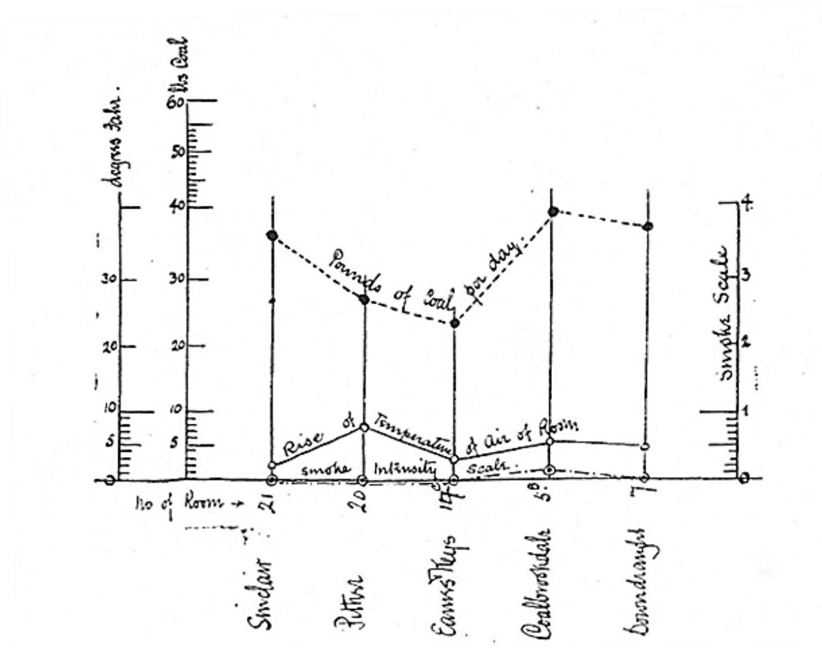
Figure 26: Results from testing of fireplaces showing rise of air temp, smoke intensity, and pounds of coal burnt (Smoke Abatement Society 1906, 182).
