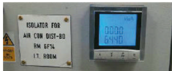
Figure 4. Dedicated energy metering of the A/C plant helps identify exact annual usage and allows more accurate assessment of its overall performance.
