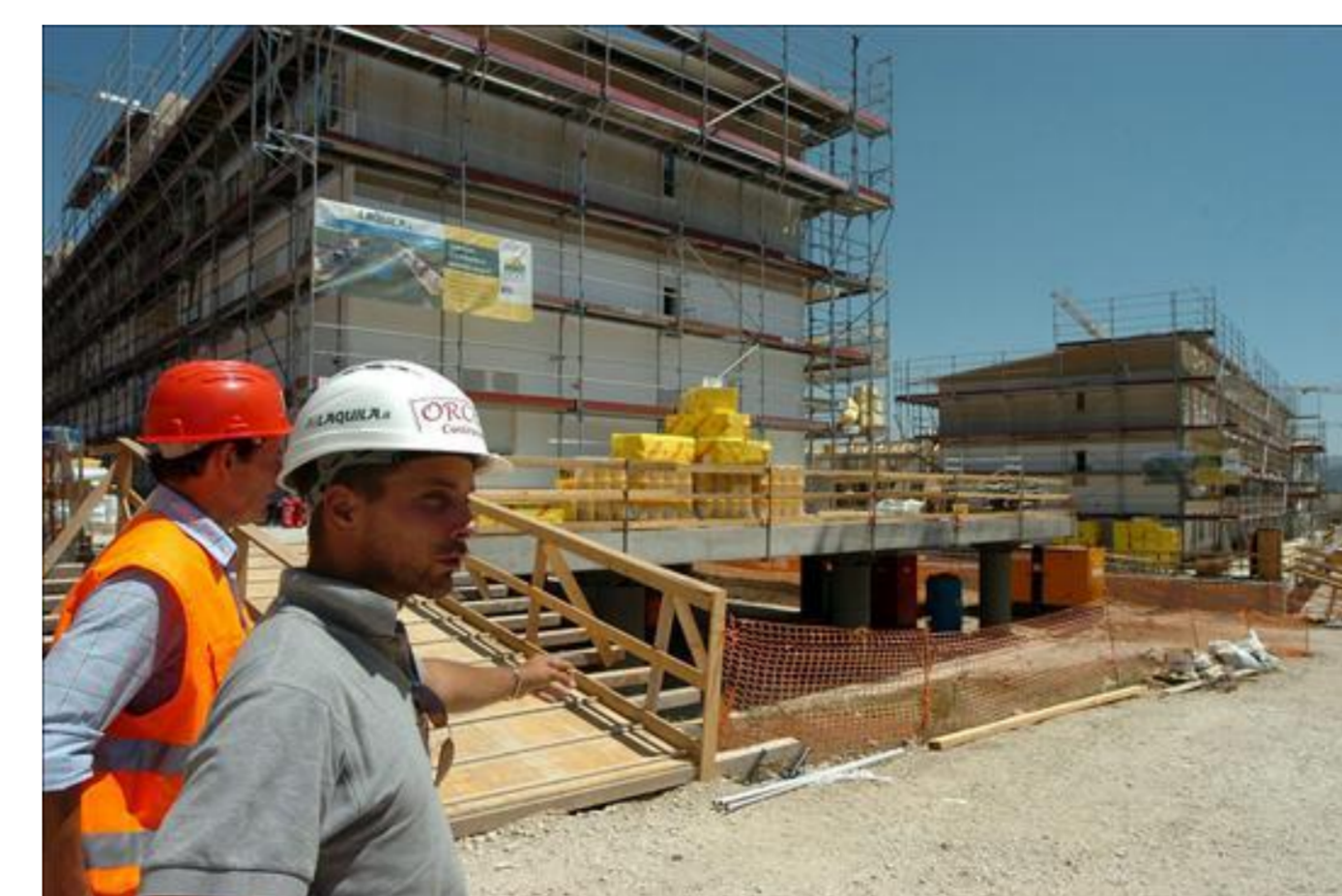
Reconstruction activities in L'Aquila (Italy). Source: European pressphoto agency
