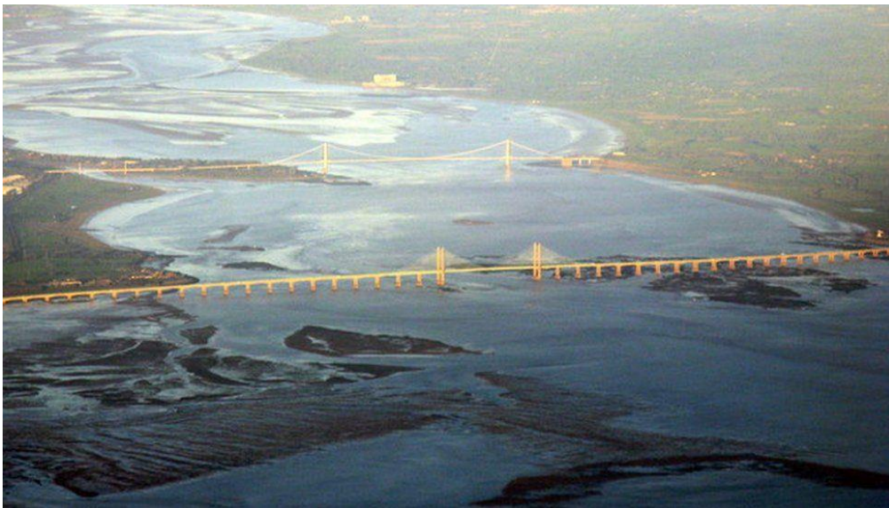
Figure 4.7. The Severn Estuary with the two Severn bridges. Photo is the property of J. Richardson.
