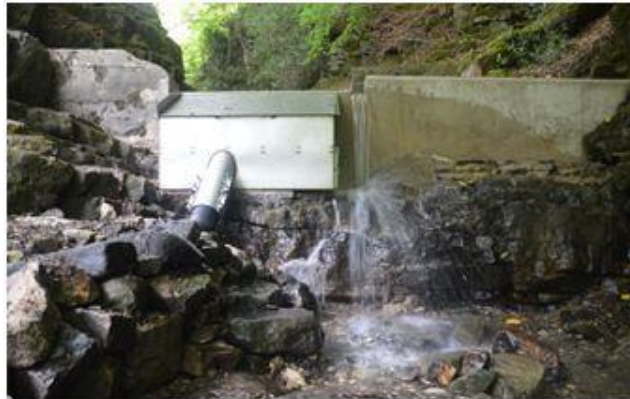
Photo 4. 4 One of the hydro schemes at Blaen Dyar site
