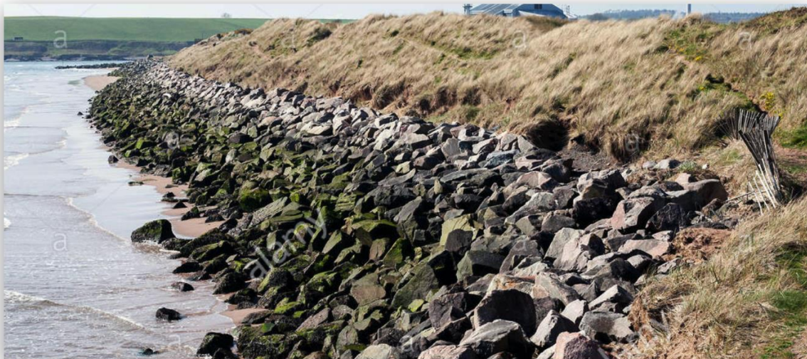
Figure 6.3.1. Example of granite boulders placed to protect unstable banking from erosion (Alamy stock photo).
