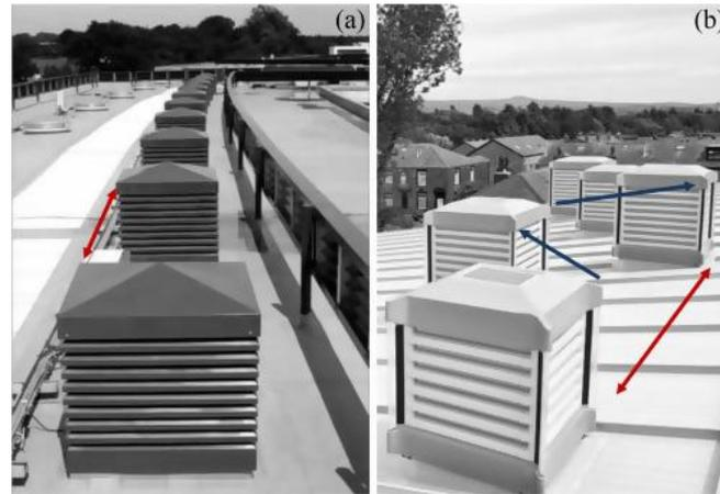
Figure 2.11: Windcatcher arrangements (a) parallel arrangement (b) staggered arrangement. Source: (Calautit et al. 2014)
