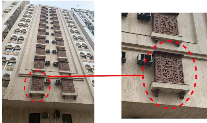
Figure 7.7: Ornamental Rawshan is constructed on a residential building in Mecca, but loses the appropriate perforation of the Rawshan's blinds
