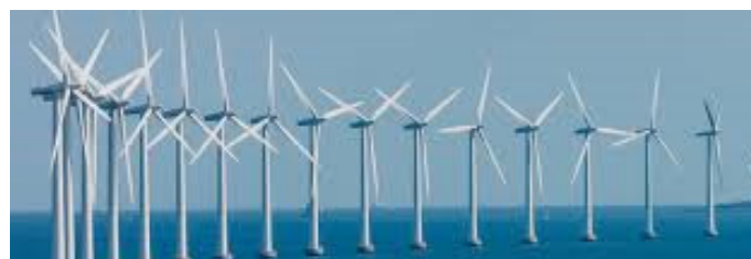
Figure 12. Wind turbine farm [82].
