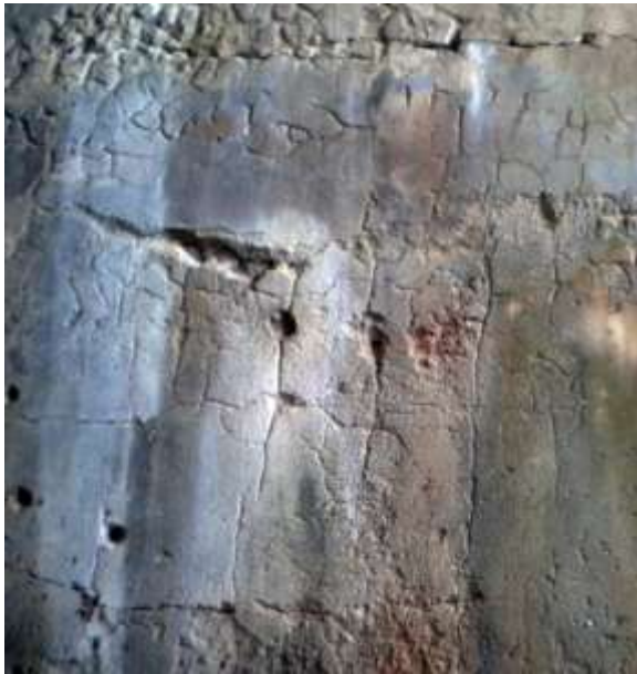
Figure 14: The wall surface, 3 rd aisle (Three-aisled cistern).
