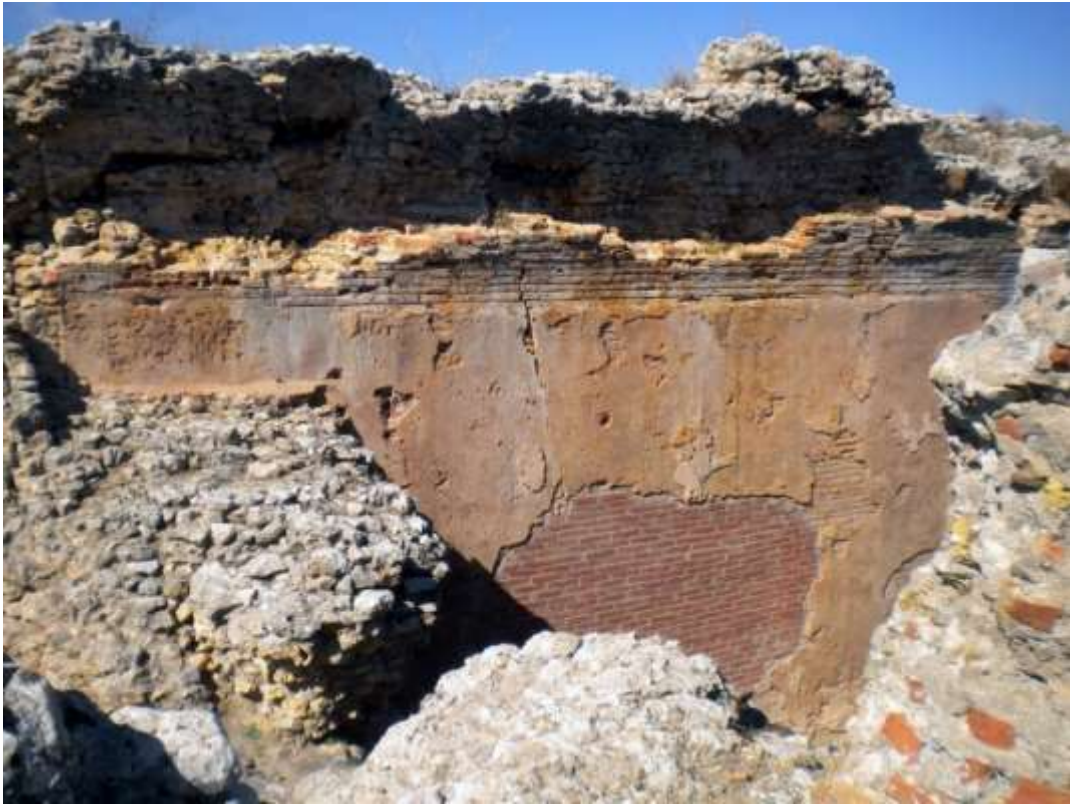
Figure 1: The gamma-shaped cistern of Aptera. The walls of the cistern are built in the opus caementicium form and the brick surface is plastered with hydraulic mortar (view from the side).
