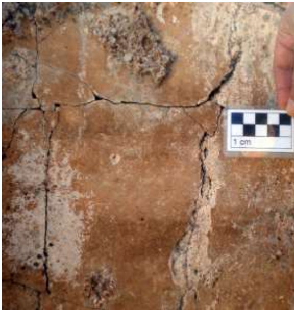
Figure 10: Sampling location on the plastered wall of the bathtub.
