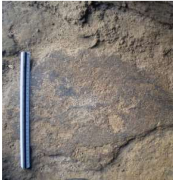
Figure 6: The surface of the low wall that separates the aqueduct from the open cistern. Dark brown-black substance is observed on the surface.
