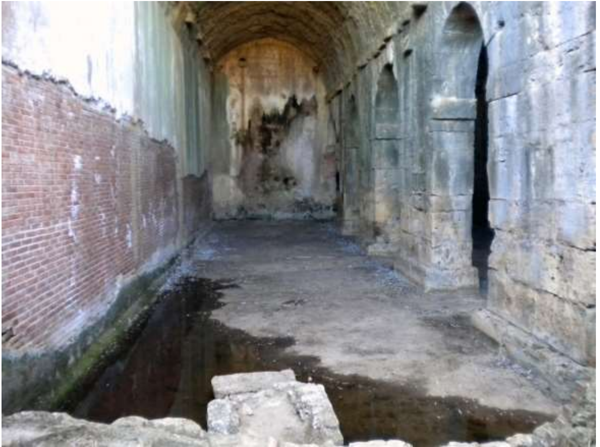
Figure 146: Apta: the three-aisled cistern (interior view).
