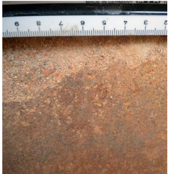
Figure 8: The plaster on the interior surface of basin 1.
