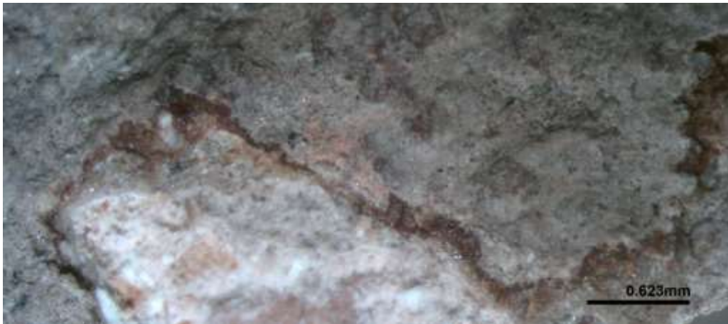
Figure 165: S3 surface layer. Resinous layer visible beneath grey soil.
