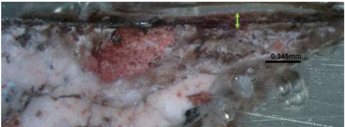
Figure 191: Cross-section of sample S15a showing a dense and thin surface layer (green arrow).
