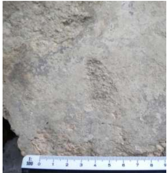
Figure 4: Detail from the surface of the stone, where the brown-black substance is observed on the mortar.
