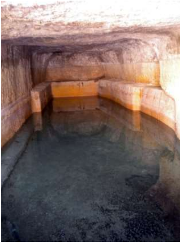
Figure 136: Polyrrhenia: the interior of the rock-cut aqueduct.
