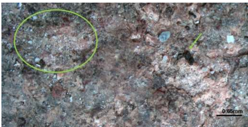
Figure 274: The surface of S27 showing black deposits and salt crystals (circled).
