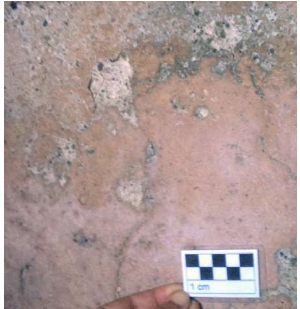
Figure 13: The wall surface, 2 nd aisle (Three-aisled cistern).
