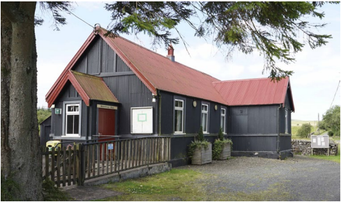
Fig. v Sheet metal building: Hermitage Library and Hall, Scottish Borders, 1910 (See Ch. 6 6.13)(OP)
