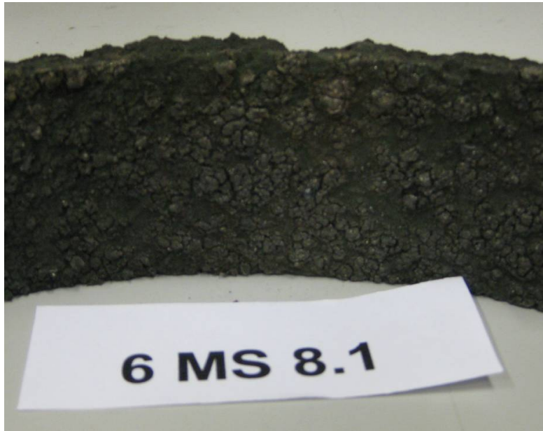
Figure 6-6 – Scale layer on inside surface of tube 6 MS 8.1
