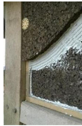
Potential Retrofit Infill materials: Wood-fibre board, sheep's wool, expanded cork and hempcrete.
