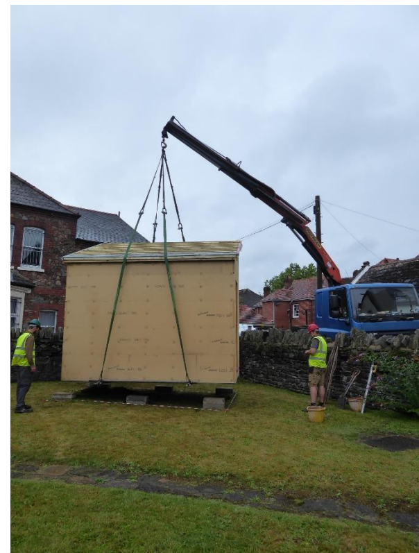
Test cell constructed by Royston Davies Conservation Builders in Leominster, with materials from Ty Mawr Lime Ltd.
