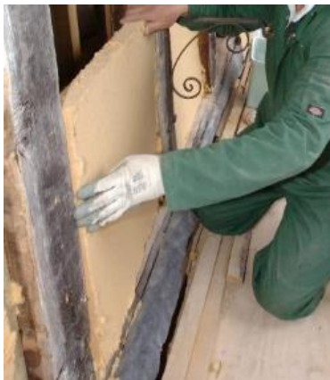
Potential Retrofit Infill materials: Wood-fibre board, sheep's wool, expanded cork and hempcrete.
