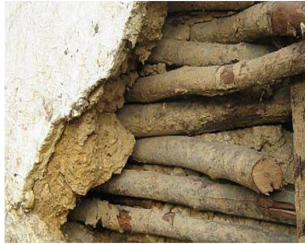
Traditional Infill materials: Wattle and daub, lathe and plaster- pargetting and fired brick.
