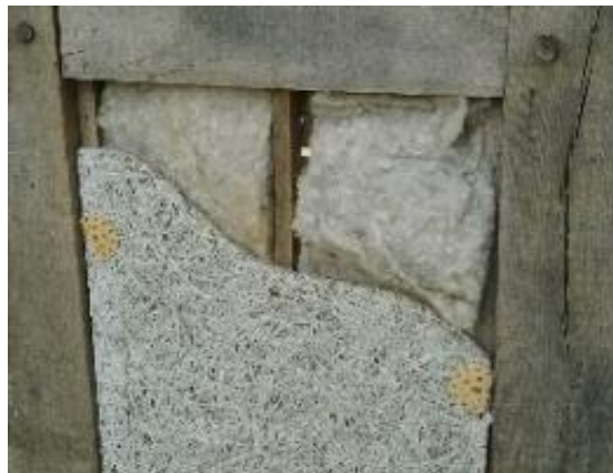
Potential Retrofit Infill materials: Wood-fibre board, sheep's wool, expanded cork and hempcrete.
