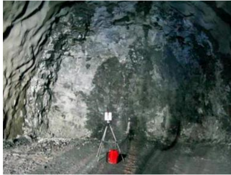
Fig.6 LiDAR scanning of a tunnel face with a diameter of 10m in Oslo, Norway [41].
