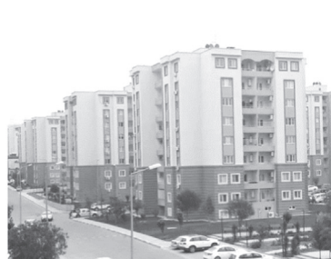
Mass construction of multi-family buildings
