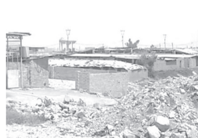
Informally self-built houses
