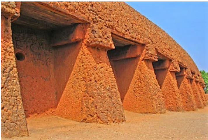
Figure 4: Traditional mud brick house, Hausa Architecture (Jehosafats 2011)
