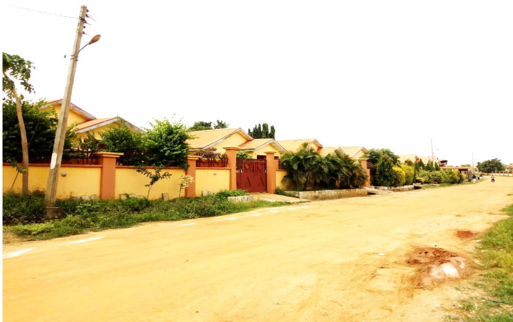
Figure 58: A section of Housing units in the Estate
