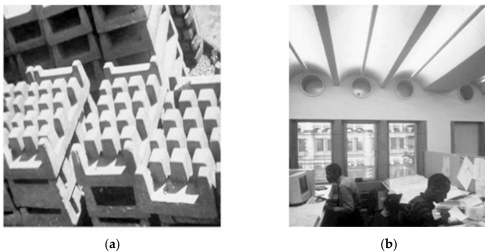
Figure 10. (a) Ecological concrete ventilated floor slabs and (b) vaulted ceilings.
