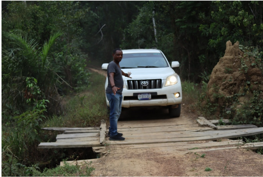
Picture 2: Plank Bridge to/from Geipa Town, Nimba County
