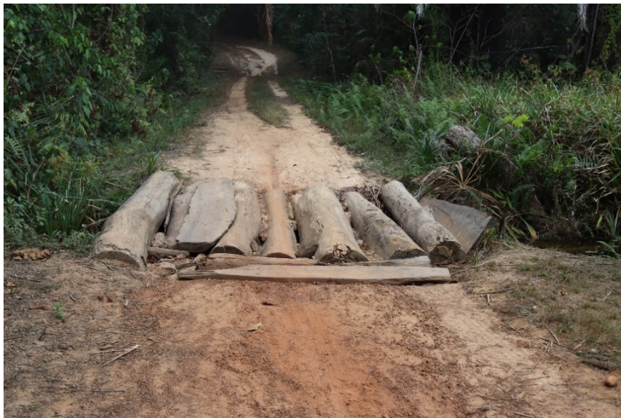
Picture 1 Log/plank Bridges enroute to/from Geipa Town, Nimba County
