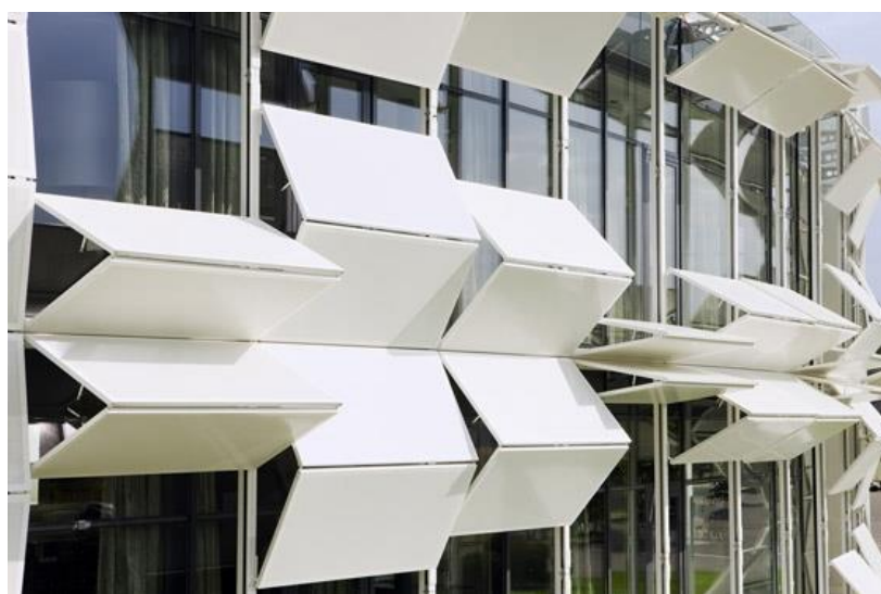
Figure 2.10: Example of a responsive façade, the Kiefer Technic Showroom.
