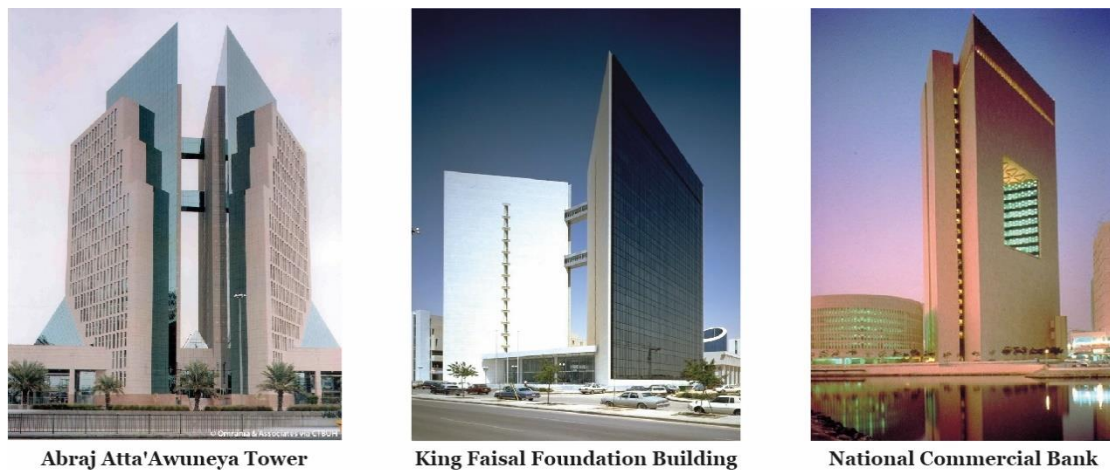
Figure 1.6: First phase of constructed tall building's structure in Riyadh.
