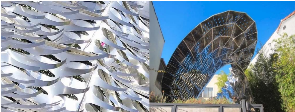
Figure 2.9: Example of smart façade, the Bloom Project.
