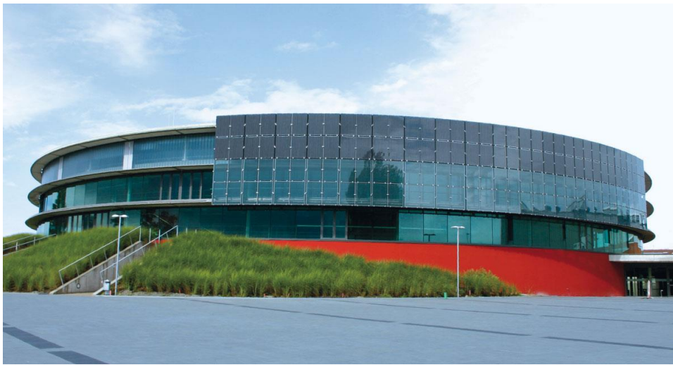
Figure 2.8: Example of movable façade, the EWE Arena in Hamburg.
