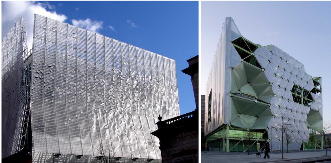
Figure 2.2: Examples of active façades the Children's Museum of Pittsburgh (left), and the ICT-Media building (right).
