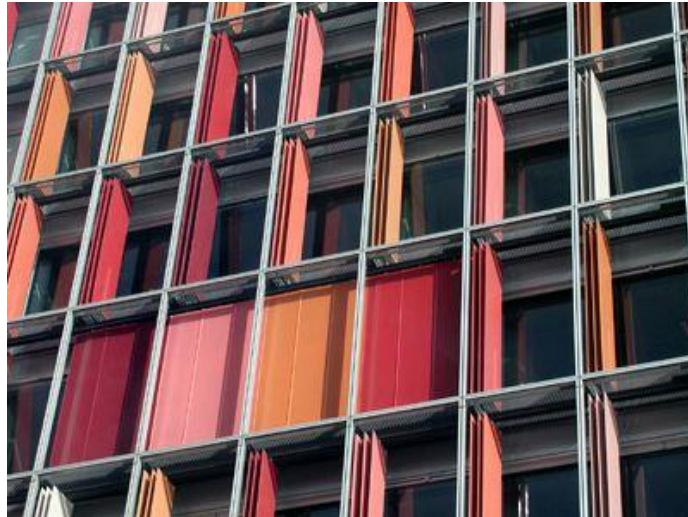
Figure 2.6: Example of an intelligent façade, the GSW Headquarters building in Germany.
