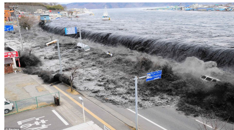
(c) Tsunami over-topping wall, Miyako Japan 11 th March 2011. Image Mainichi Shimbun/Reuters
