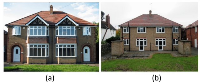
Fig. 3. Houses adopted from [9] to verify the numerical model in IES VE: (a) front; (b) rear.
