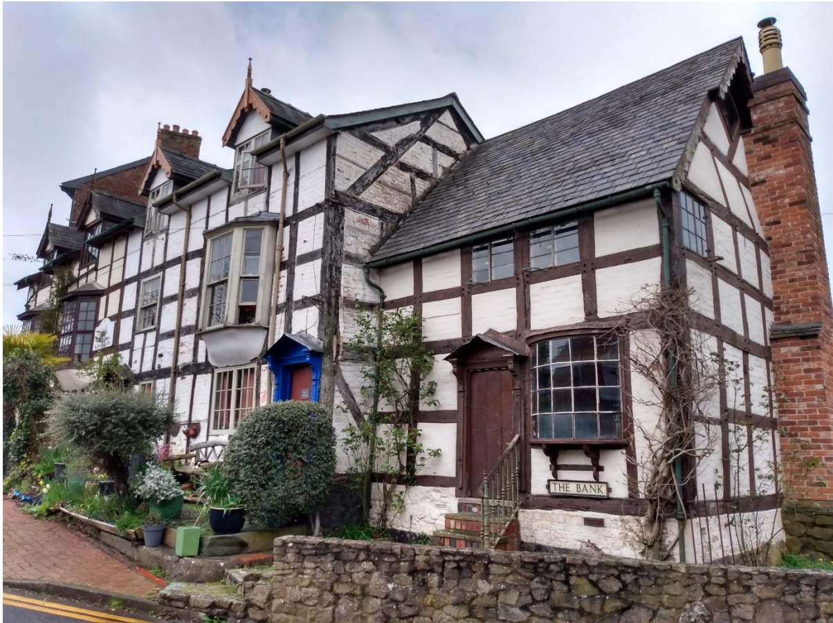
Figure 1. 17 th century timber-framed buildings with 19 th century alterations, Newtown, Powys, Wales (Source: author, 2024).
