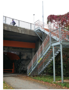
Figure 8. The stairway linking the neighbourhood and Klostergata. Photo: O.H. Hagen.
