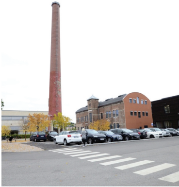
Figure 3. Reconstruction of chimney and old industrial building. Photo: O. H. Hagen.
