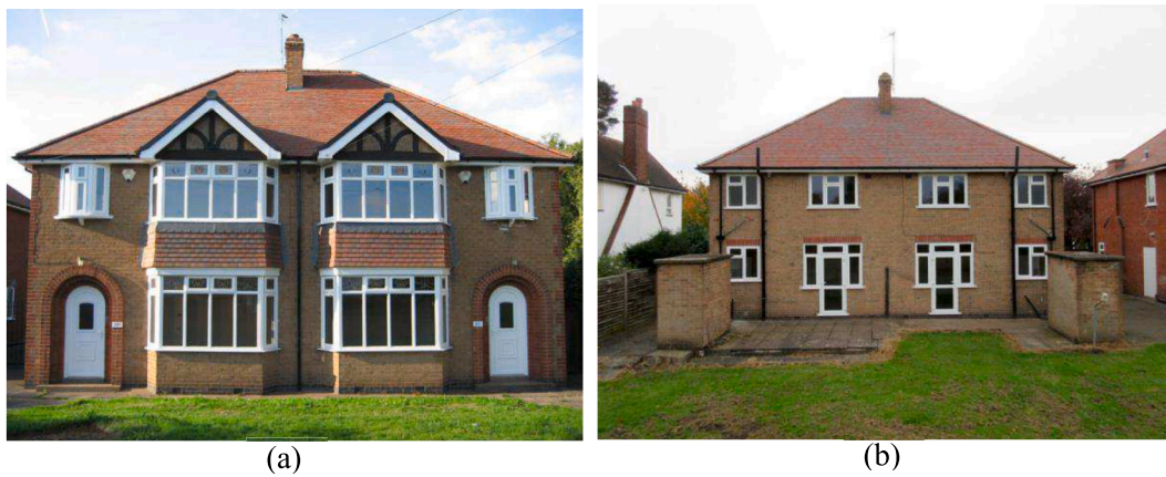
Fig. 11. Front view (a) and rear view (b) of the matched-pair houses used in the experiments in [37]. The house on the left in (a) was used for verification of the house model presented in this paper.
