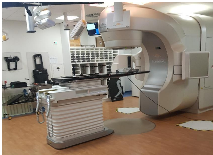
Photo 2. Radiotherapy treatment room with treatment machine (linac) and couch.
