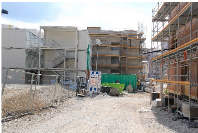
Photograph 4. Construction site for new residential buildings (300).
