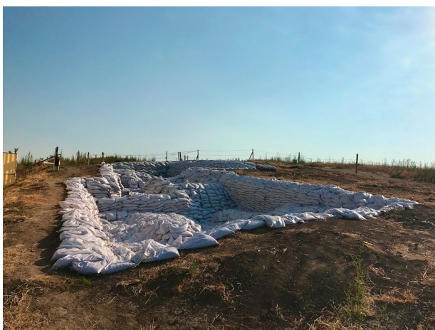
Figure 1. External trench, Çatalhöyük, Turkey. This trench is at the top of the Neolithic mound and is in an area exposed to wind and water runoff. The trench was first lined with geotextile, and then polypropylene agricultural woven sacks filled with backdirt were systematically layered within the trench.
